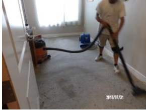
Prepping the floor in a resident room before the new carpet.
